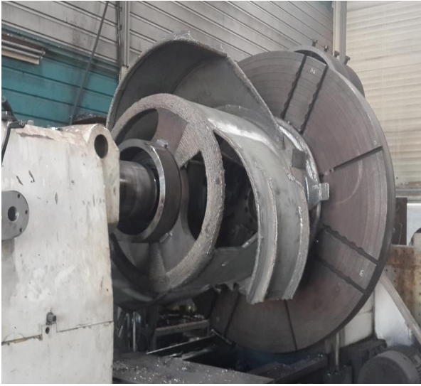
Repair CSU Inlet Feeder
